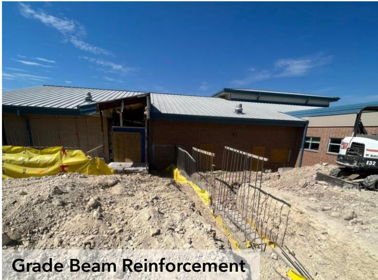
Grade Beam Reinforcement
